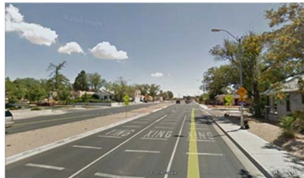
Photo 7. Bike Striping and Signage at Silver/University
